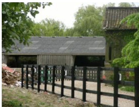
Disused former farm buildings at Home Farm
