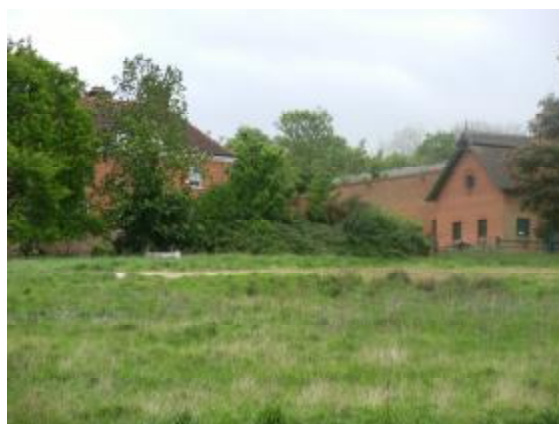
Little Copped Hall (left) with model farm building at Home Farm (right)
