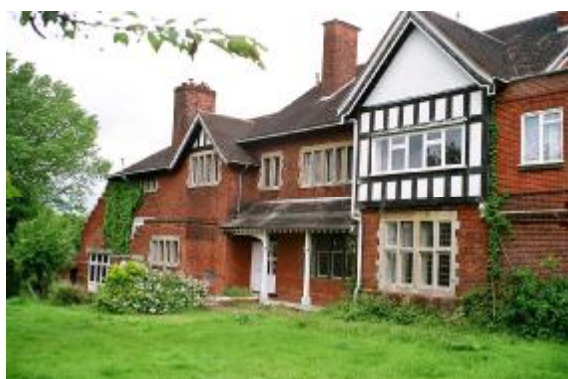
Griffins Wood House
