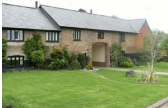
Nos. 1 & 2 The Hall Barns, Copped Hall
