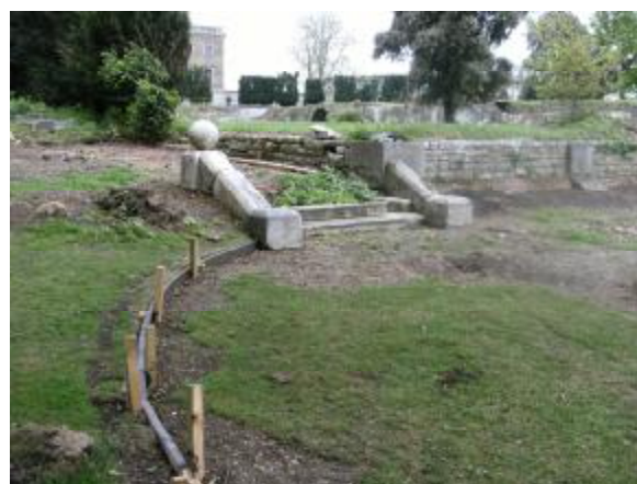
Garden restoration in progress
