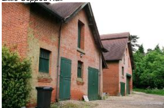
The Hayloft and Stables (model farm buildings) at Home Farm, Little Copped Hall
